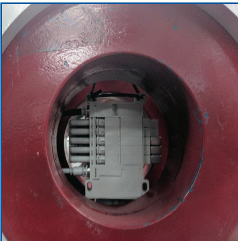
Solenoid valve manifold sandwiched between coil faces. Photo: US ITER/ORNL
