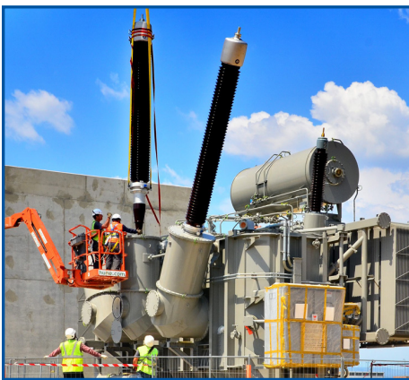
Installation of bushings for high-voltage transformers. Photo: ITER Organization
