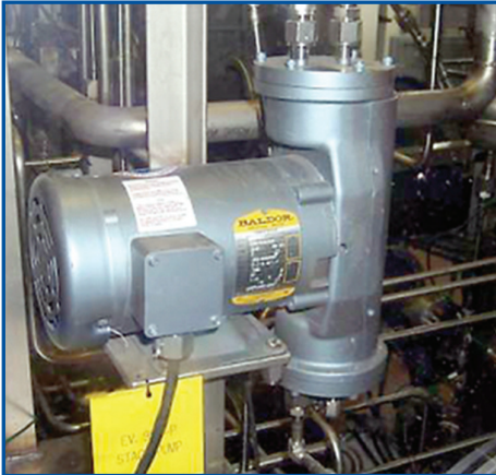
Metal bellows pump. Photo: US ITER
