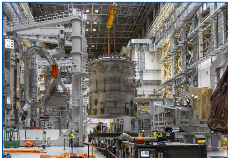
A view of the ITER assembly hall as an auxiliary cold box is transferred for positioning into the tokamak building. Photo: ITER Organization
