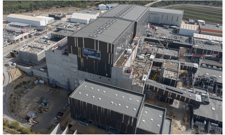
The ITER tokamak complex in October 2024. Photo: ITER Organization
