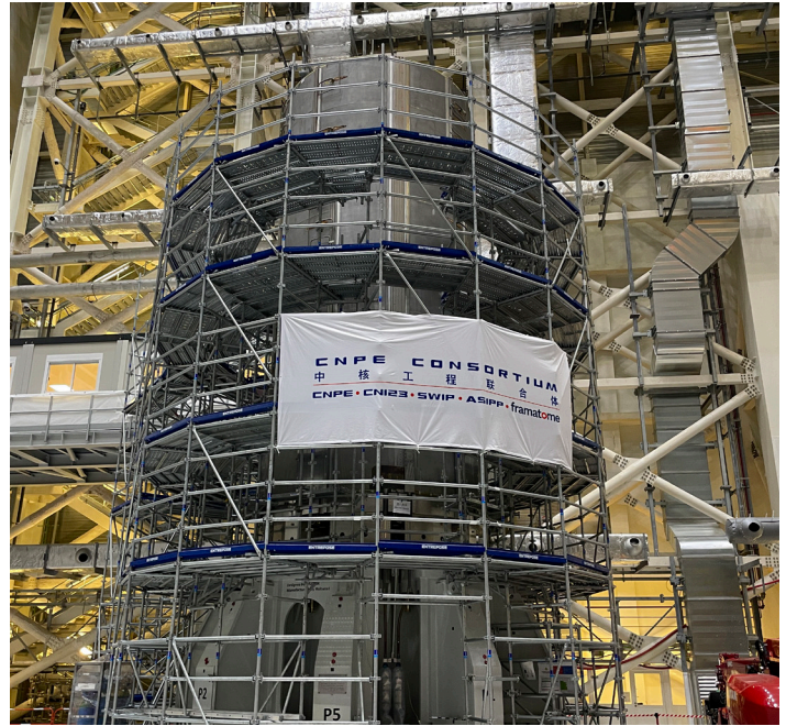
US ITER is delivering the “heart of ITER,” the superconducting central solenoid magnet. The first four magnet modules are stacked for assembly. Photo: US ITER
