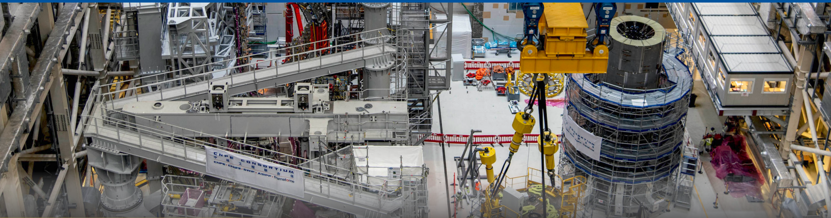
Numerous activities are underway in the ITER Assembly Hall, including vacuum vessel sector (left) and central solenoid assembly (right). Photo: ITER Organization
