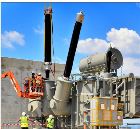
Installation of bushings for high-voltage transformers. Photo: ITER Organization
