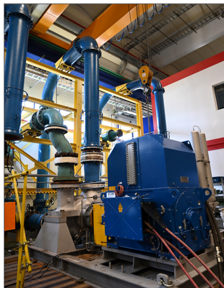
Assembly is complete for this primary pump of the vacuum vessel heat transfer system. Photo: US ITER
