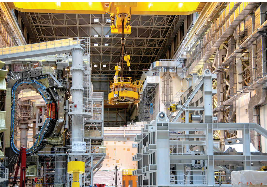
A U.S.-provided central solenoid magnet module (center) is positioned for assembly inside the ITER facility. Photo: ITER Organization
